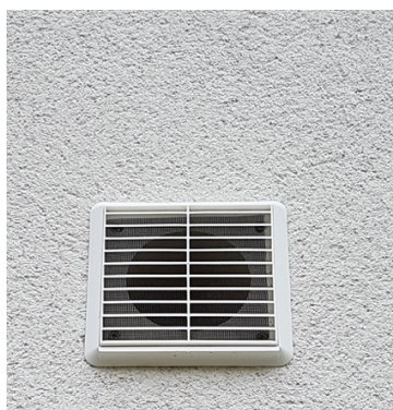
Photo 3- External louvres to kitchens should not have insect mesh.
