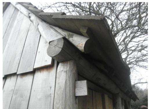
Sweet chestnut posts were used to construct Conkers office in 2002, and had no trouble proving their strength, they have proven perfectly durable and they are fully exposed.
