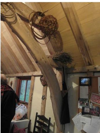
Pierre has a small demonstration building constructed from elm, with poplar roof lining boards, wattle and daub infill panels and a wide range of wicker baskets and chopping boards for sale.
