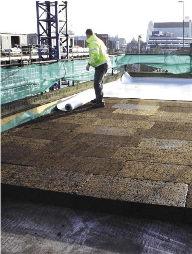
The cork board being laid over the existing asphalt roof with the new waterproof membrane being laid over it.
