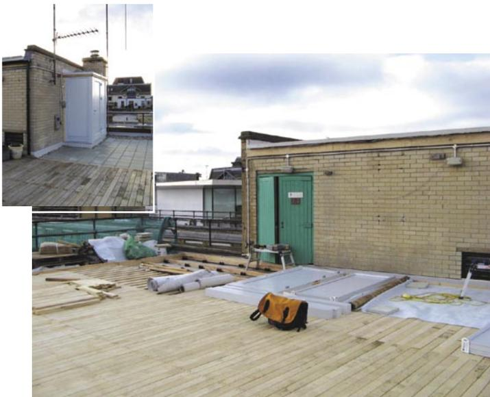
Terrace decking being laid on protective geotextile and rubber pads. Larch bearers support sweet chestnut decking. Inset: new porch for easier access by staff.
