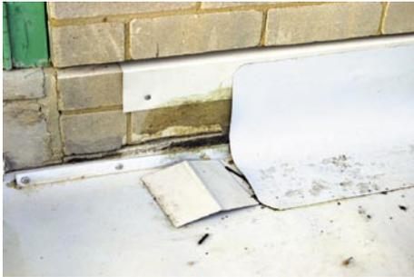
Membrane edge detail with retaining bar to maintain tightness of covering. Metal coated flashing dressed into wall, membrane welded between flashing and main roof covering.
